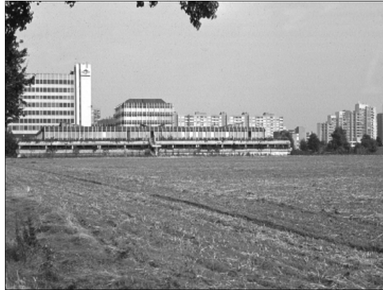
Figure 12 An urban border without positive ecological functions (Darmstadt, Germany). Biotope mappings can help to find sufficient solutions for designing an urban border.
