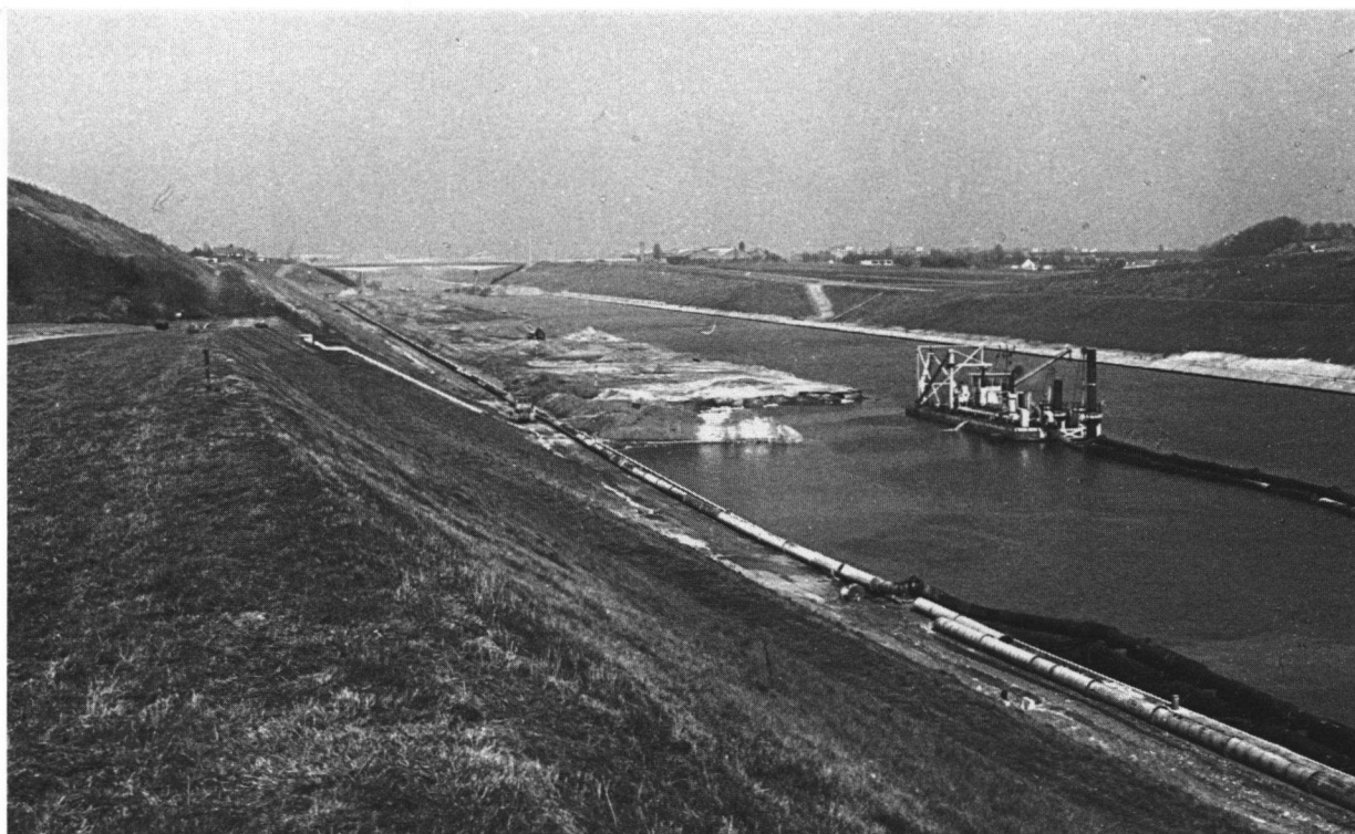
Fig. 2. The Albert Canal at Riemst, province of Limburg, Belgium, looking North, with the Veldwezelt bridge in the background.
